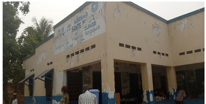
Nkufulu Health Centre before renovation
