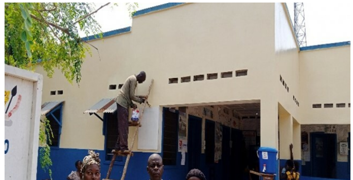
Nkufulu Health Centre after renovation
